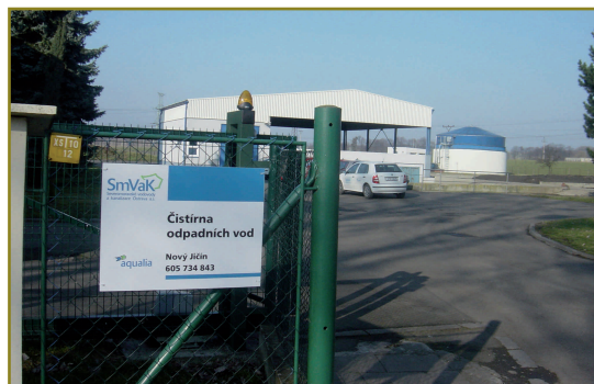
Nový Jičín water treatment plant, Czech Republic, managed by SmVak.
