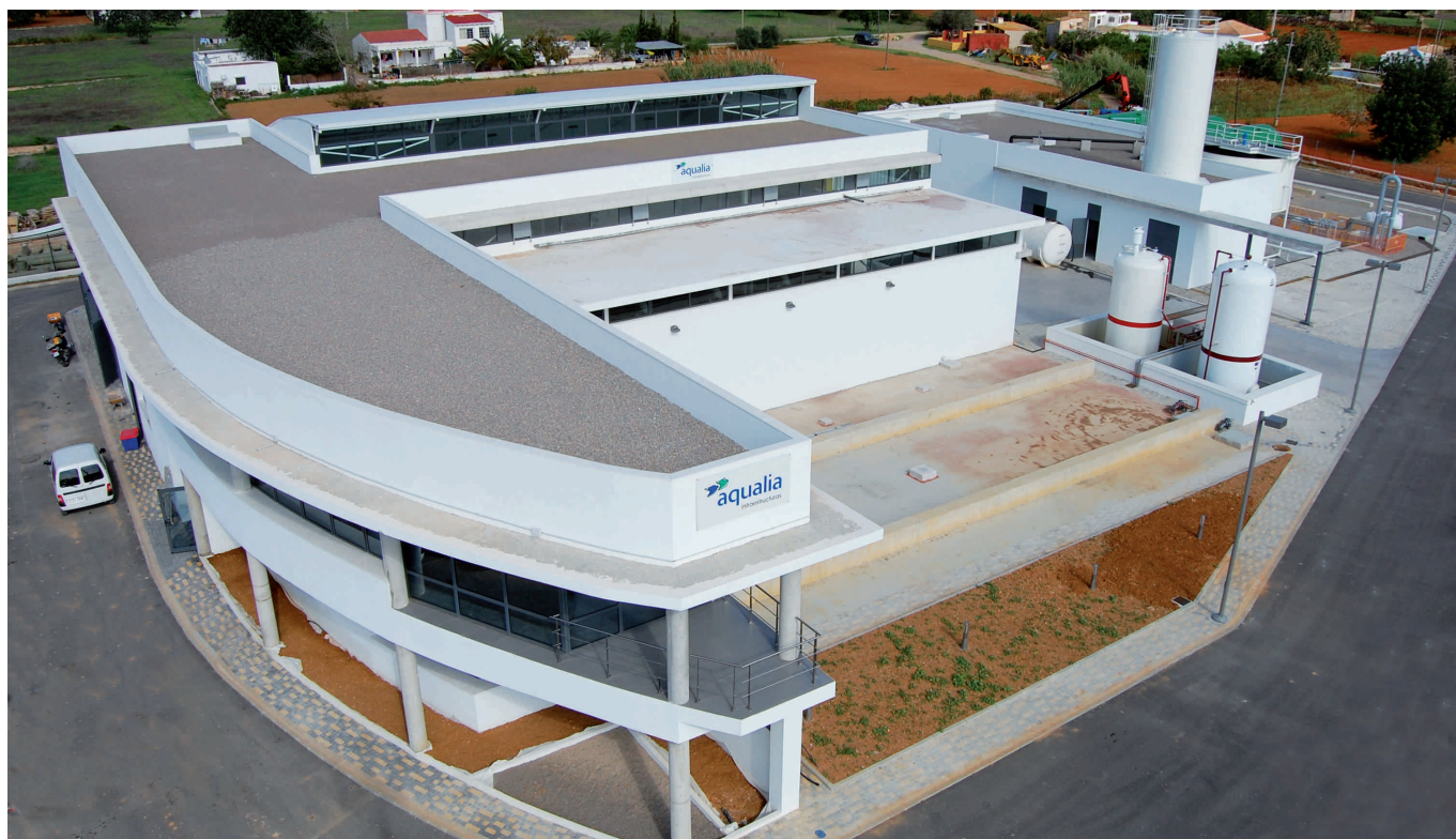
Desalination plant in Santa Eulalia (Ibiza).
