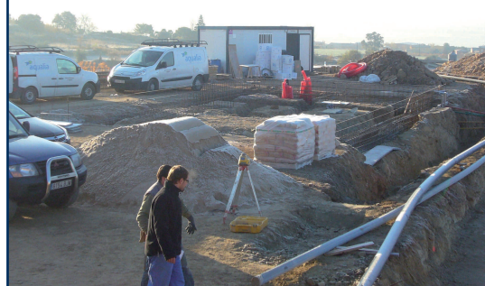
Construction work at the Penelles' DWTP, Lleida.
