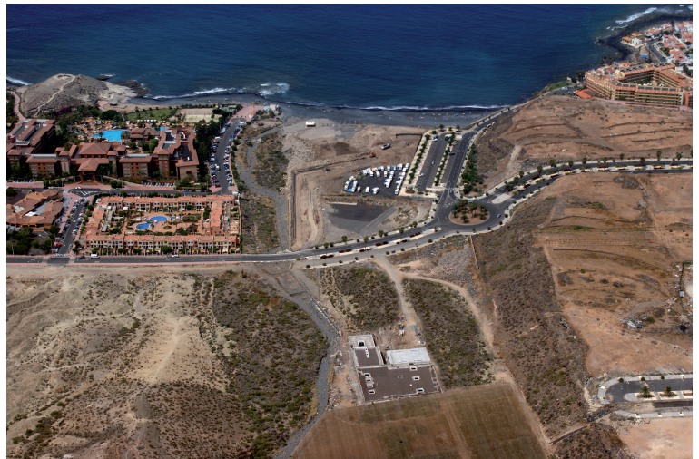
Adeje's plant reduced the visual and acoustic impact to a minimum.
